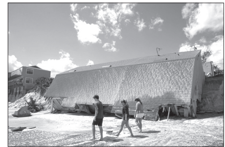
Class of 1955: Hurricane Irma damage, St. Augustine Beach
