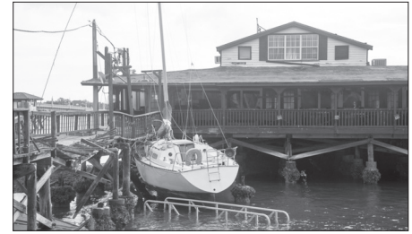
Class of 1955: Hurricane Irma damage: City of St. Augustine, Restaurant on the harbor in downtown
