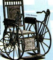
The first practical wheelchairs provide new 1760 mobility for those unable to walk. Early models of wheelchairs have three wheels and hand cranks to propel the chair forward.
